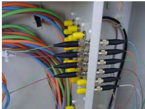
Fiber Optic Cable Terminations
